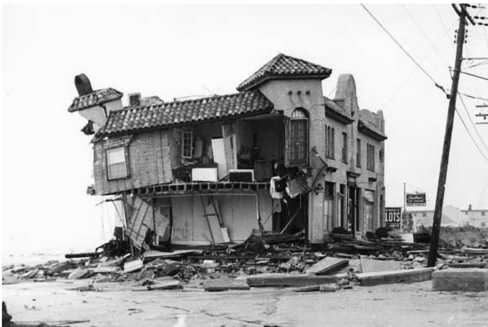
Shown here is the building at 100 West Brigantine Avenue. The storm washed out the foundation and the north end of the building collapsed. Below, a boat that rode the tide inland from the bay came to rest in front of the island diner.
